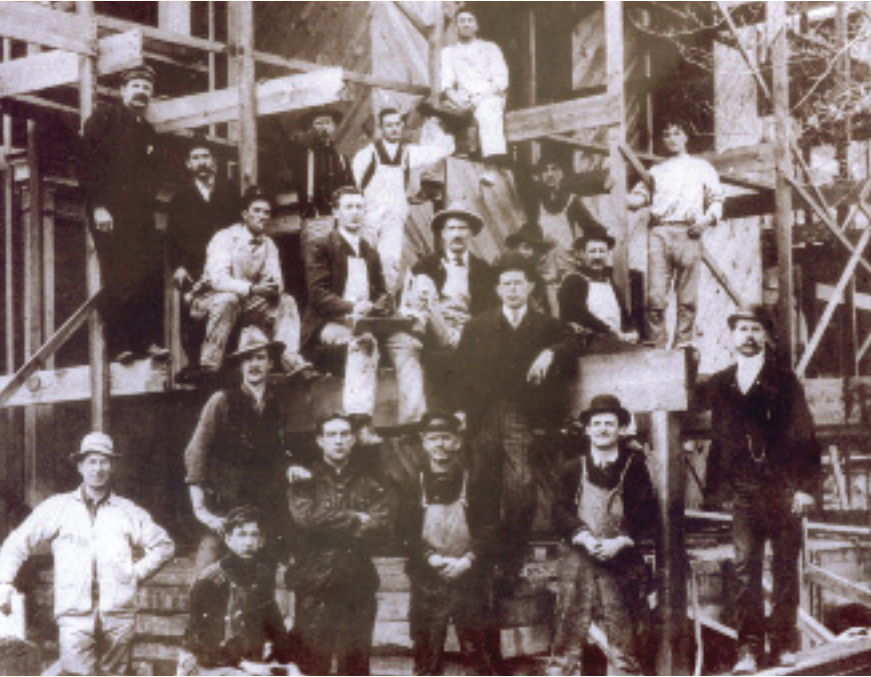
A group photograph of workers engaged in building the Kuser mansion shortly before its completion in 1905. (Private Collections)
